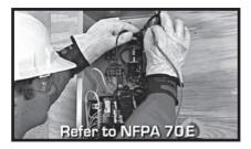
When all emergency circuits have been moved to the transfer switch, close the main breaker to restore utility power and make sure utility voltage at the transfer switch is correct. Refer to NFPA 70E for the safety equipment required when working inside a live transfer switch.
